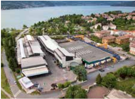
OFFICINE NICOLA GALPERTI E FIGLIO S.P.A. FORGING PLANT I - ITALY
