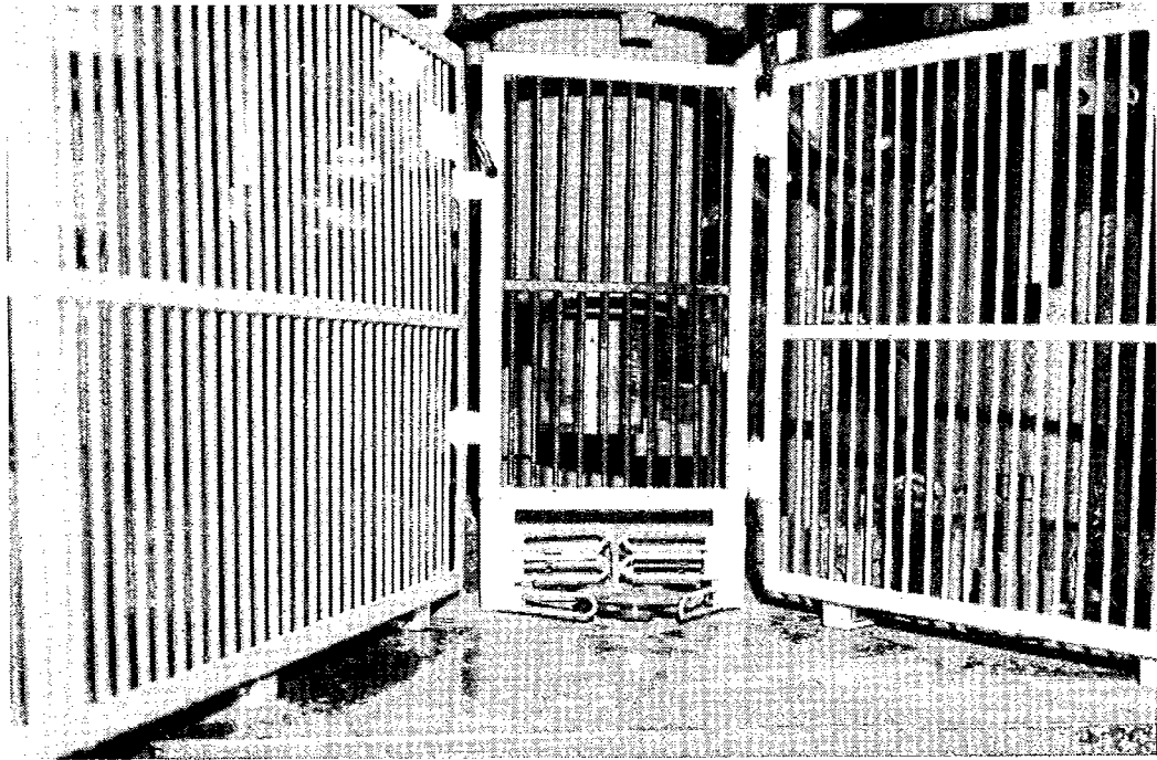
Illustration 11 A Typical Barrier Gate Device
